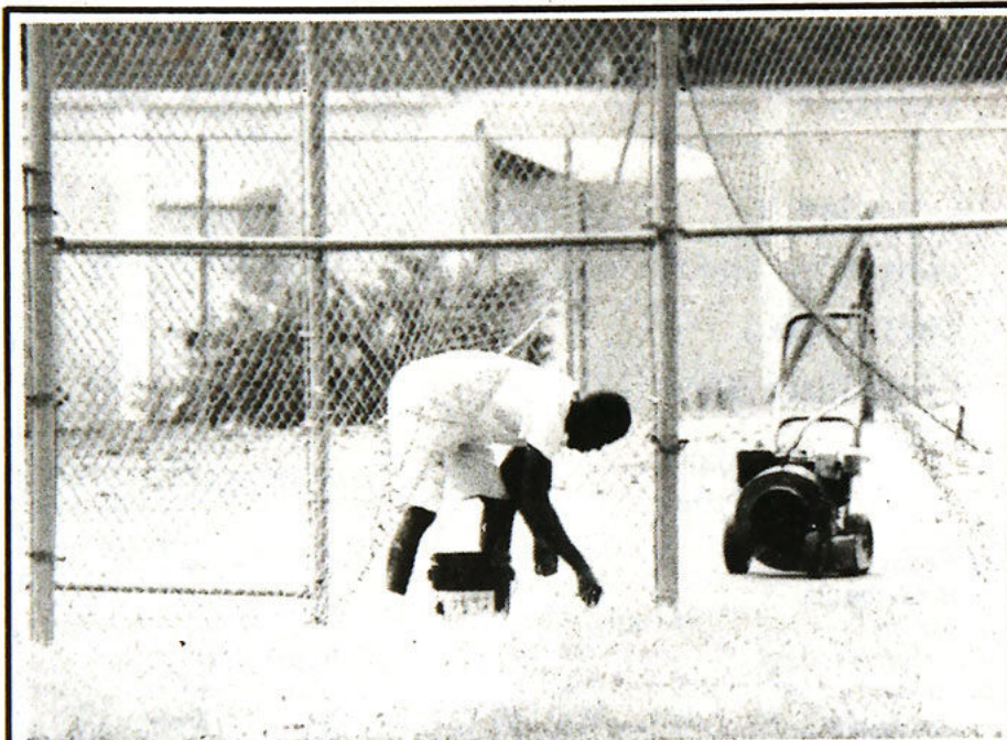
A worker prepares the court for resurfacing. Picture By Daniel Eckert
