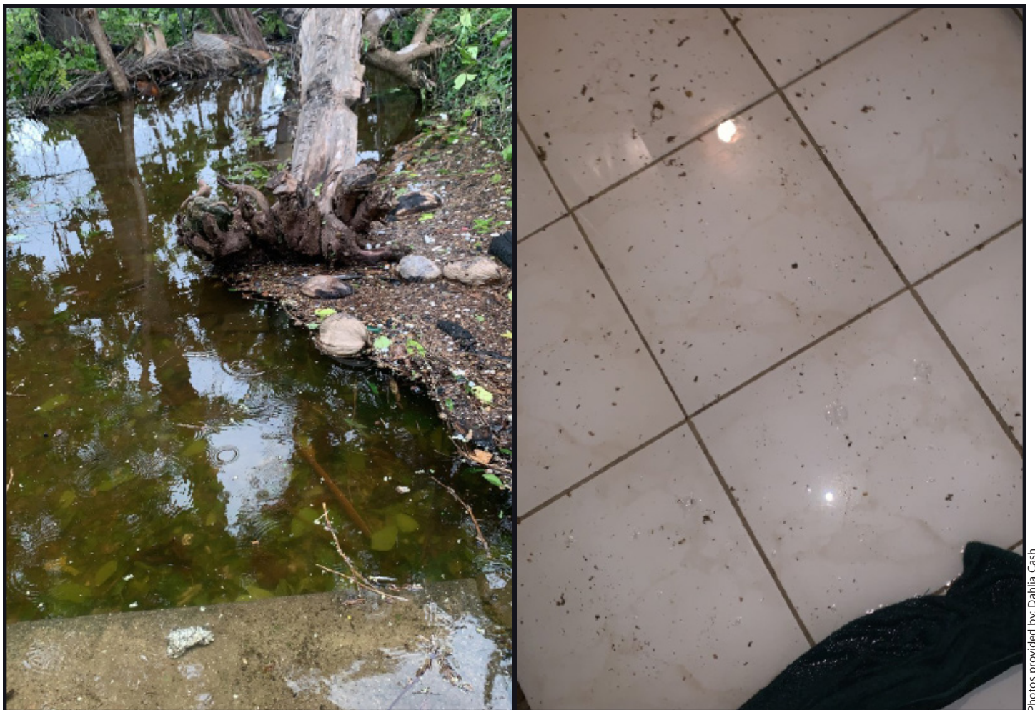
Cash's home was directly impacted as trees in her yard were rooted up by the gusting winds. Water from the outside poured into her living room as the outer bands of the storm whipped the capital of The Bahamas.
